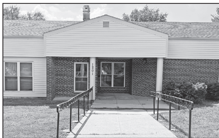
West Central Community Action will combine its offices at the former Sunshine 'N' Rainbows building later this summer. (Nick Johansen/The Red Oak Express)
